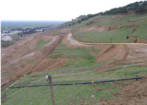
Fig. 3: Gas and water pipelines crossing a tension crack of the landslide, with the village of Devechi in the background
