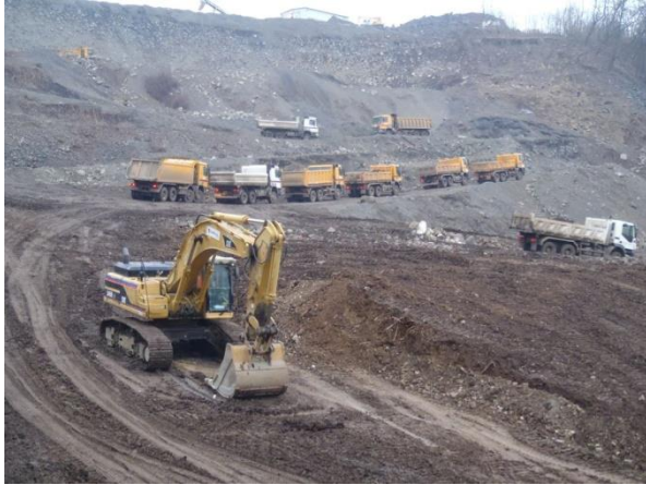
Fig. 6: Excavation of 80.000 m 3 in the upper part.
