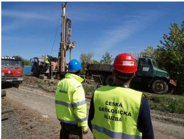
Fig. 4: Site investigation – borehole HV103.
