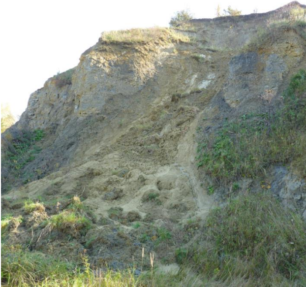
Fig. 5: Rock pillar affected by openings of cracks
