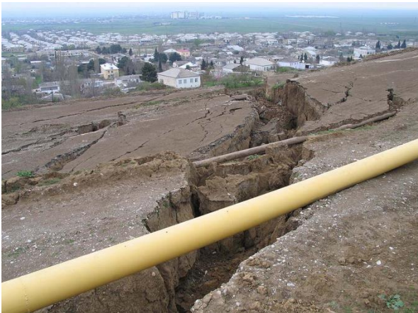
Fig. 2: Overall view of the landslide
